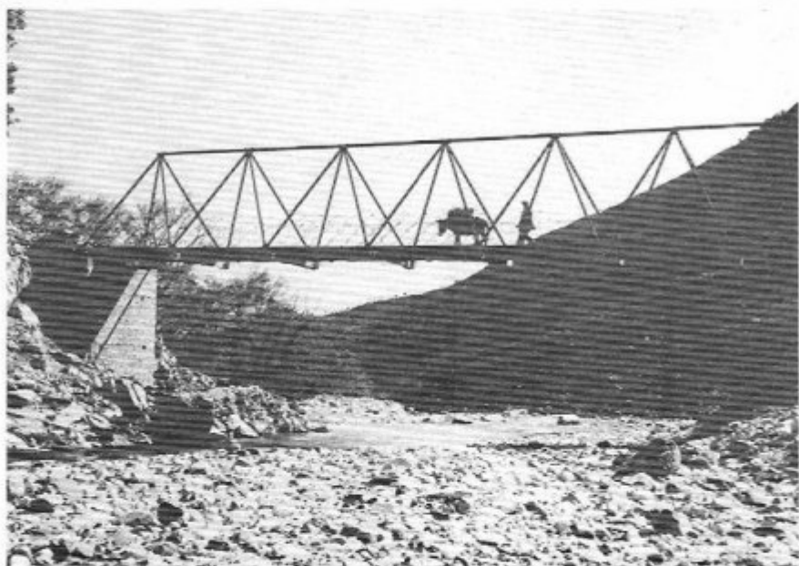
Koniska. Steel bridge
